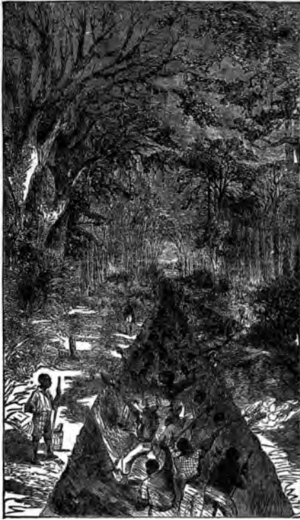
Digging a canal across the peninsula on the Louisiana side of the river, in order to carry the army and supplies below Vicksburg, but which proved a failure. Located by Brigadier-General Williams.
